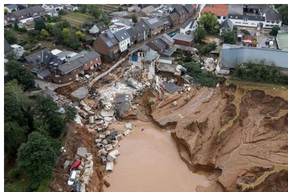
Flood in Germany (2021)
